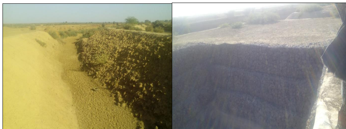
Drain principal (DP)
