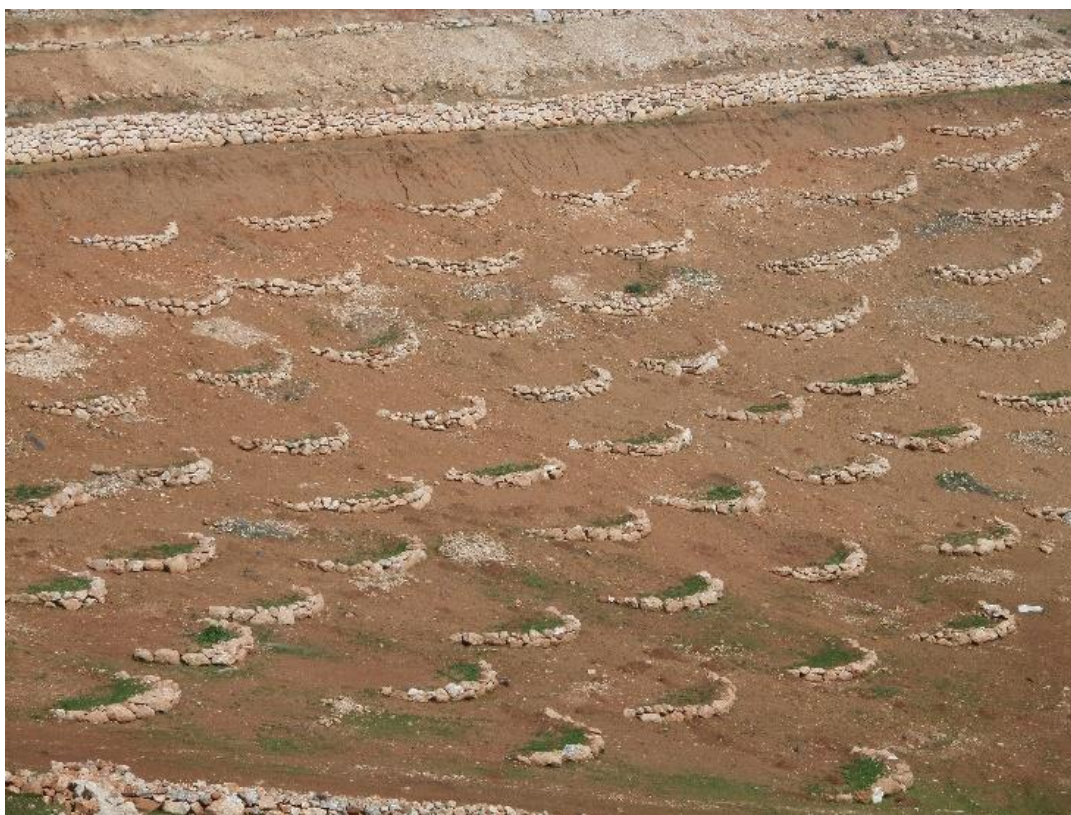
PHOTO 5.1: RAIN WATER HARVESTING EYEBROW TERRACES. (PHOTO COURTESY ARIJ)
