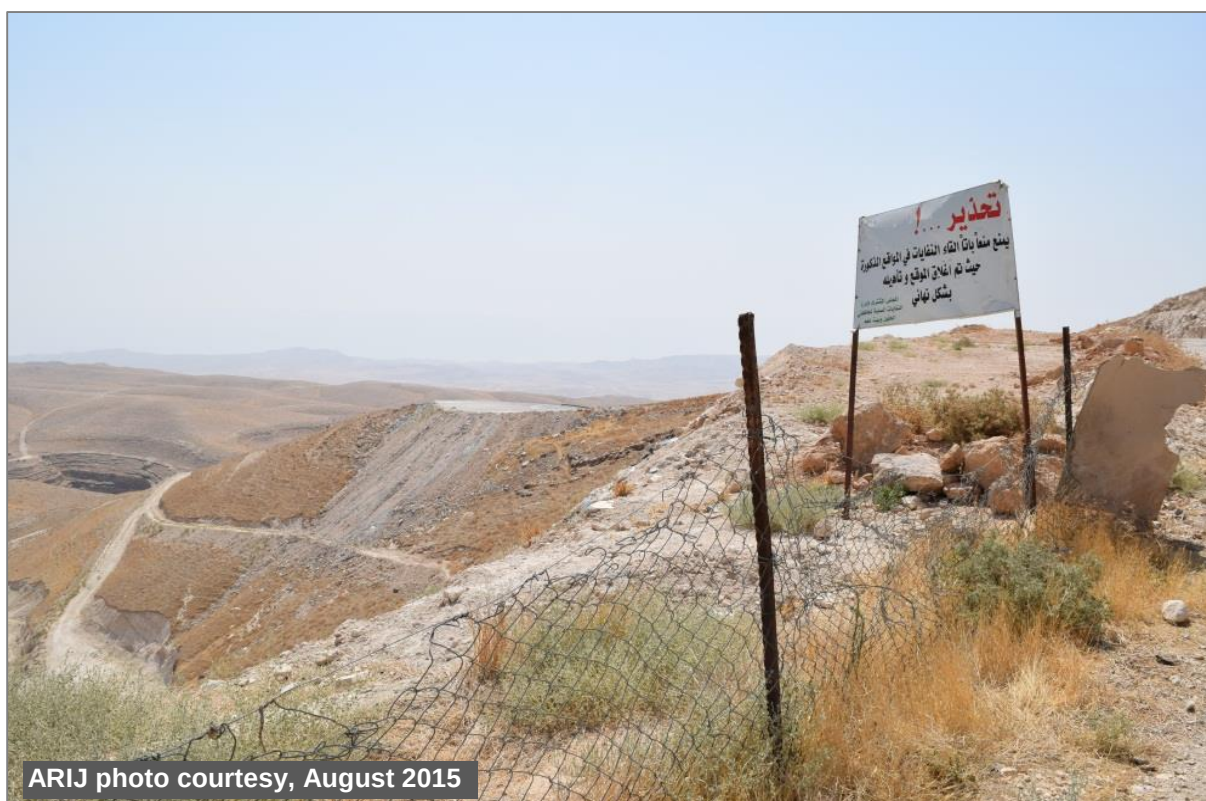
PHOTO 3.2: AL UBEIDIYA RANDOM DUMPING SITE AFTER REHABILITATION
