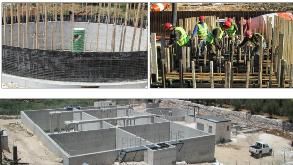
PHOTO 2.3: SAIR WASTEWATER TREATMENT PLANT DURING CONSTRUCTION PHASE
