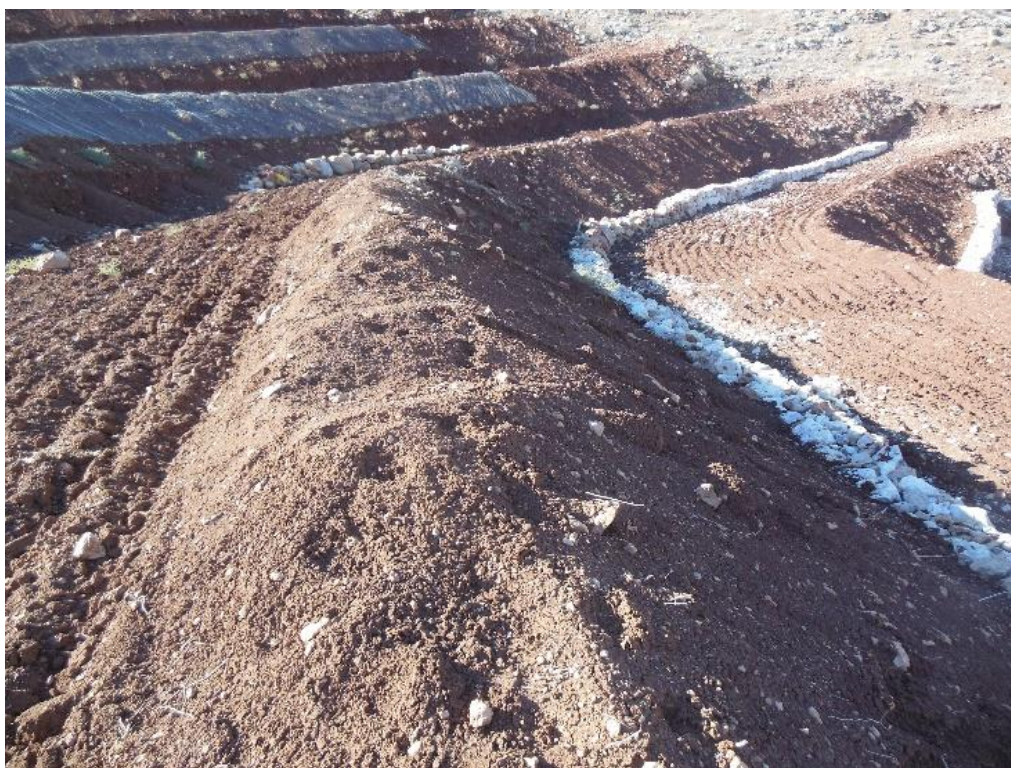
PHOTO 5.2: RAIN WATER HARVESTING CONTOUR BENCH TERRACES (PHOTO COURTESY ARIJ)
