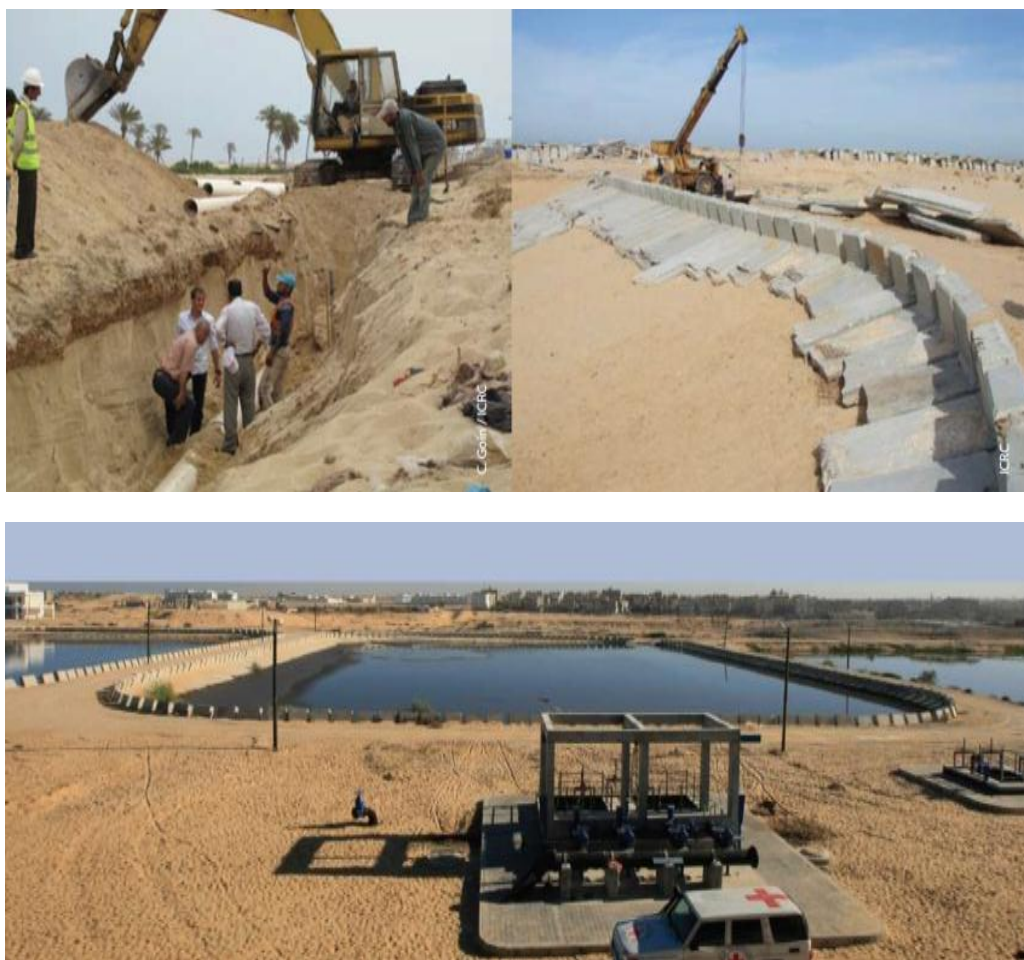
PHOTO 2.6: RAFAH WASTEWATER TREATMENT PLANT UNDER UPGRADE TO INCREASE ITS CAPACITY AND ENHANCE ITS EFFLUENT UTILIZING RECYCLED FRAGMENTS OF DEMOLISHED WALL SEPARATING GAZA AND EGYPT. (PHOTOS COURTESY OF ICRC)
