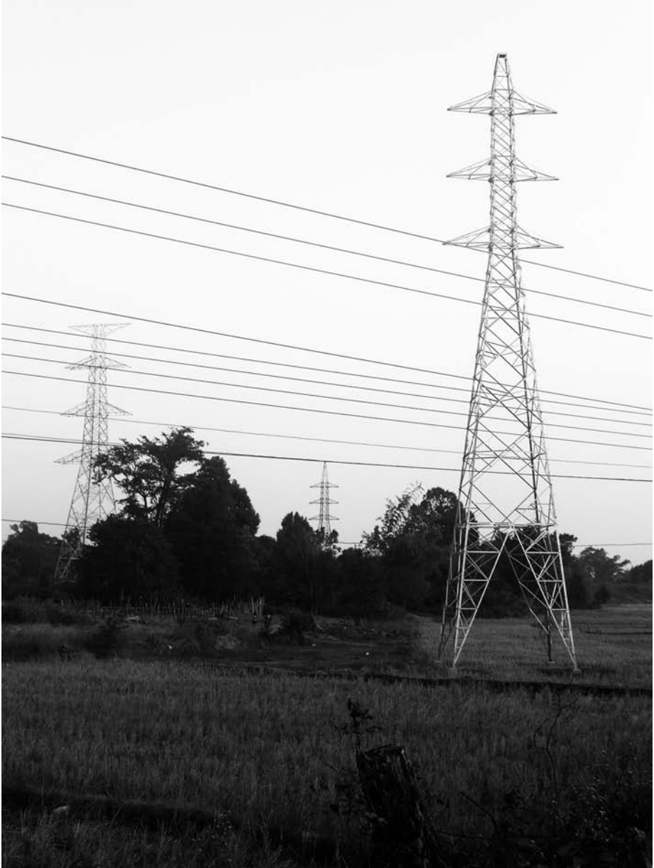
Figure 4.1 Nam Theun 2 Transmission tower
