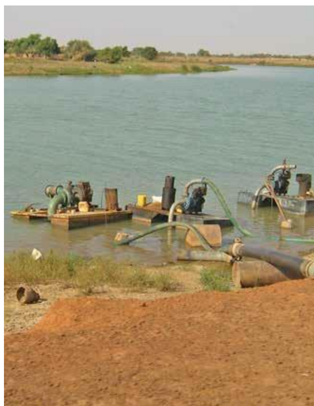
Small private pumping systems in the Senegal River Valley (Podor) © B. Vennat
