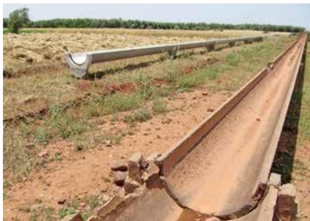
Rehabilitation of self-supporting canals - Region of Marrakech, Morocco © F. Deram Malerbe
