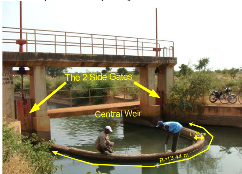
Figure 45: Dimensions of the regulator weirs
