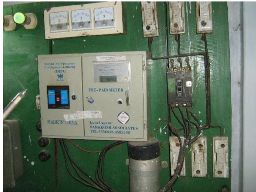
pre-paid meter install in a collect if pumping system
